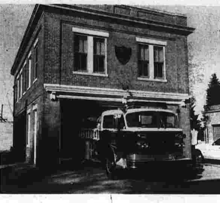
All Work Completed If the truck fits, put it in. All the work has been completed at the School Street firehouse and the new fire truck is ready for service. The door at the house was widened to accommodate it. (Herald photo by Pinto)
